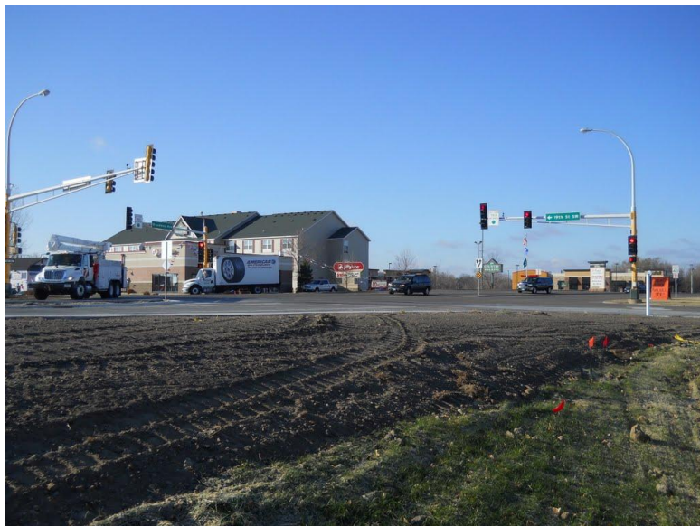
The Broadway Avenue/19 th Street intersection signal system
