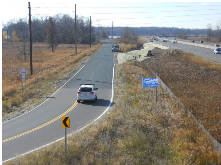
Eureka Ave. (looking south)
