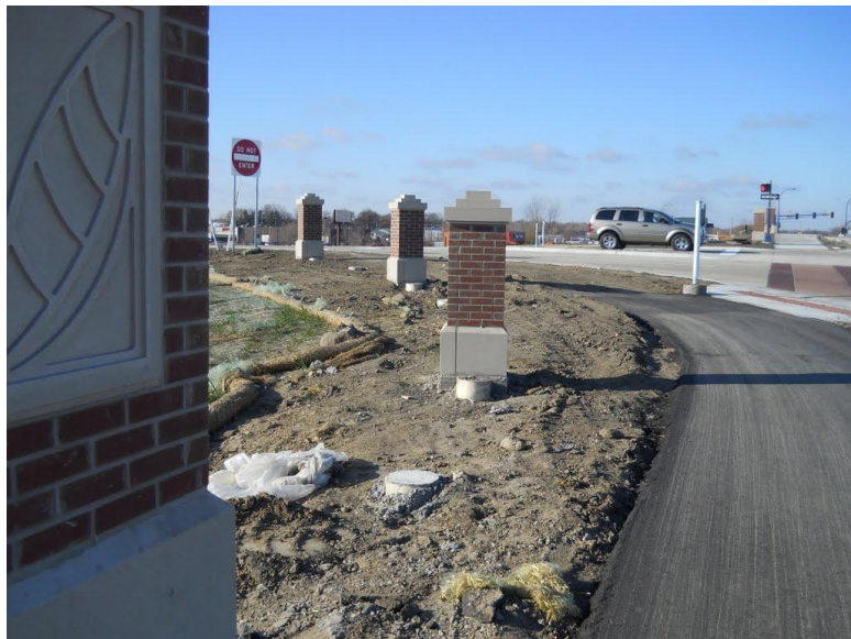
Footings for ornamental rail and monuments
