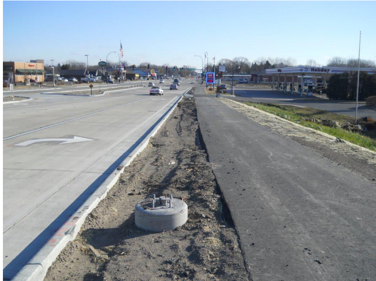
Footing for a future light pole
