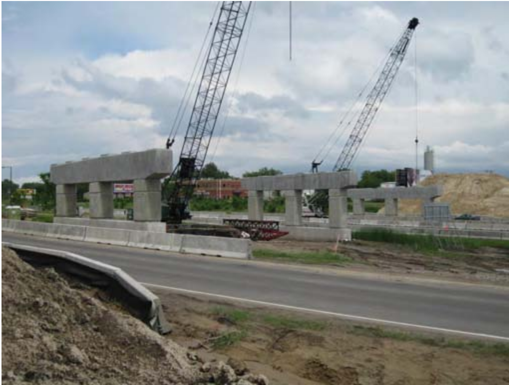
View looking east at the three completed bridge piers
