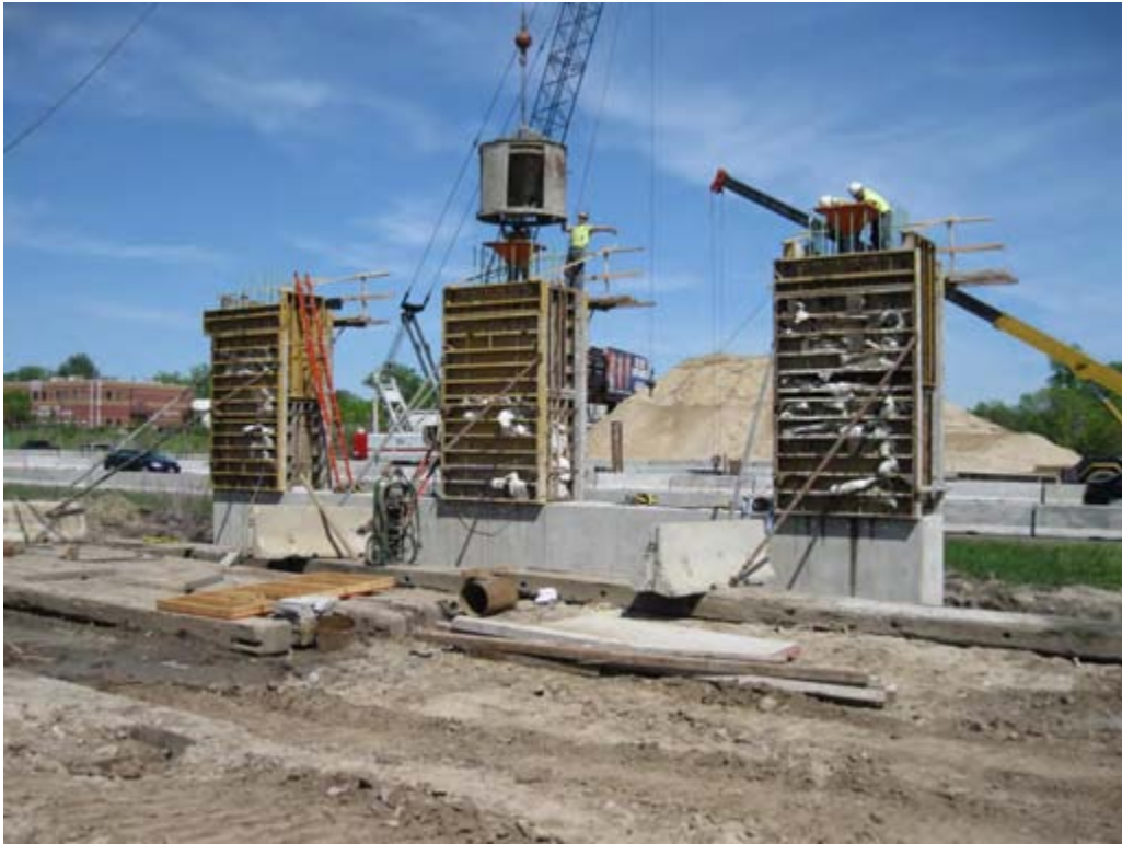
R.R. Schroeder construction workers pouring columns for pier 2
