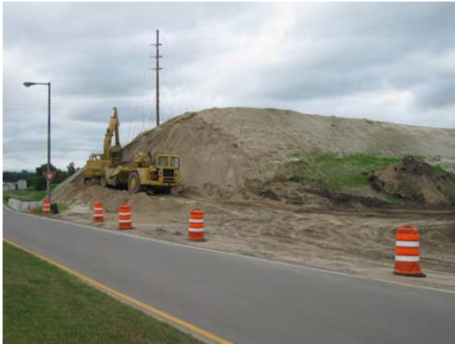
Excavation of the west surcharge
