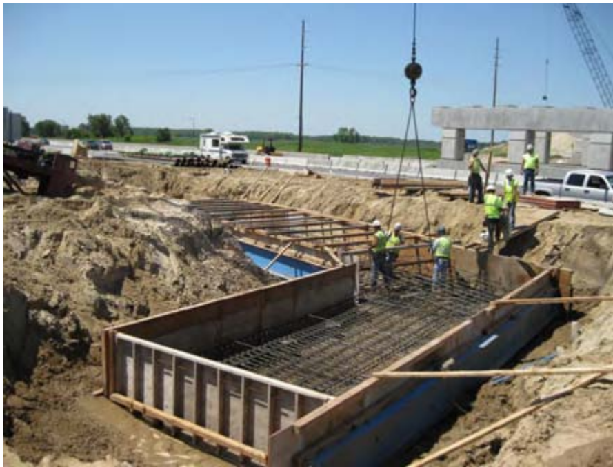
Placing of forms and reinforcing steel for the east abutment footing
