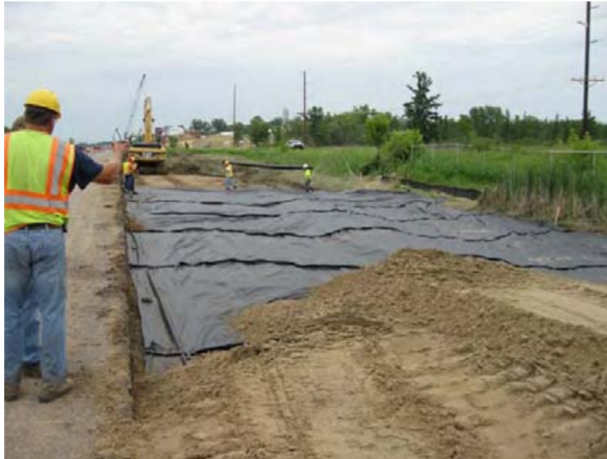
Beginning of construction for the temporary northbound off-ramp
