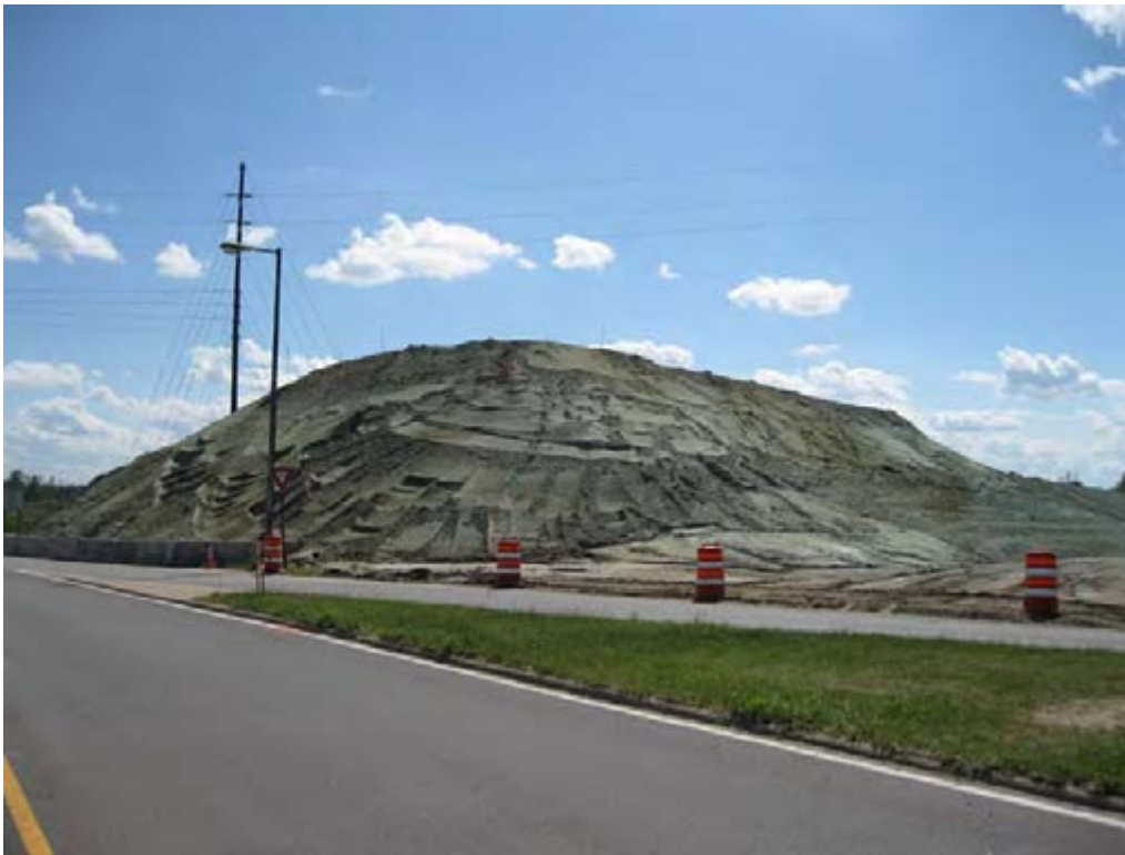
Completed surcharge on the west side
