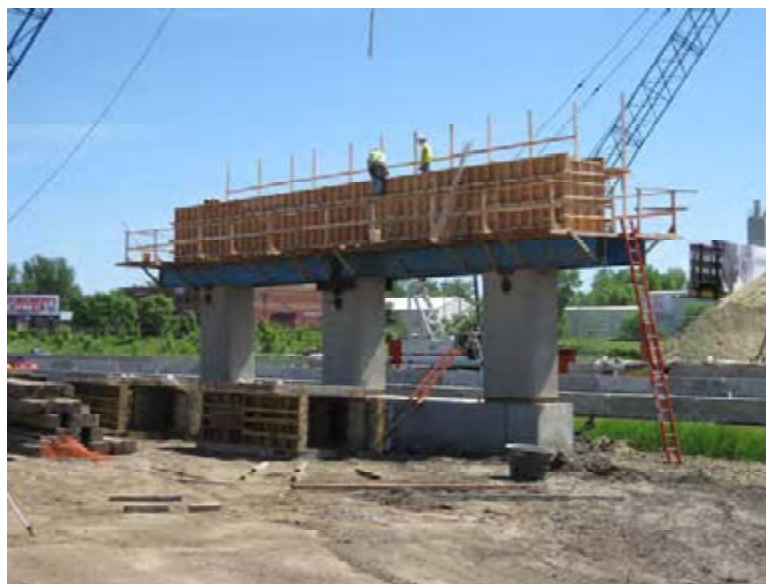
Formwork being assembled for pier 2's cap section
