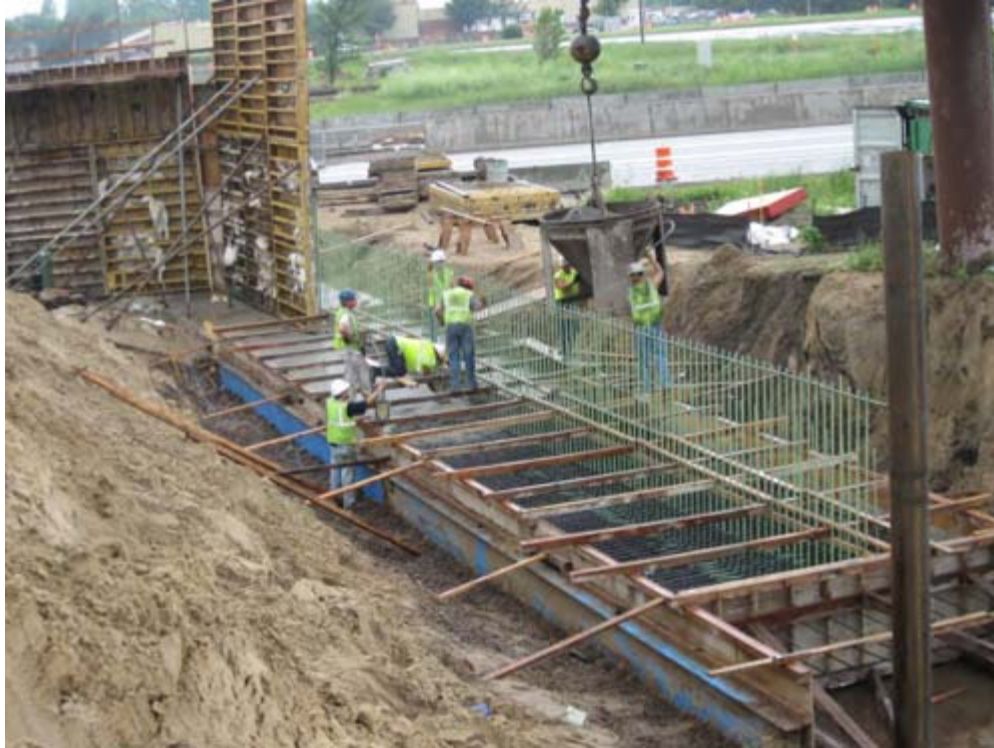
R.R Schroeder workers pouring part of the north retaining wall's footing
