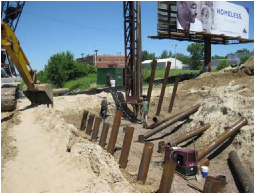
Pile driving at the east abutment
