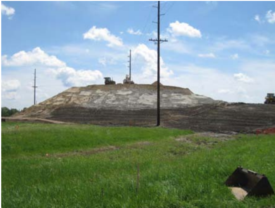
Hauling of embankment material nearing completion on the west side
