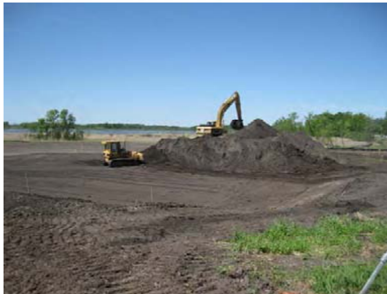
Excavation work at the west infiltration basin
