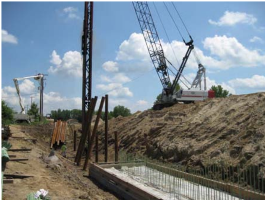
Pile driving operations for the north retaining wall footing
