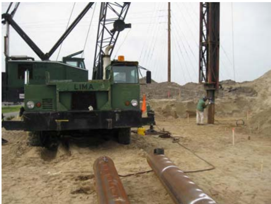
A worker welding a splice on a west abutment pile.
