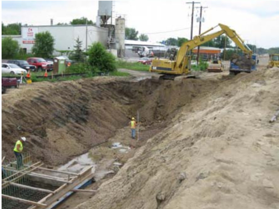
Excavation for the north retaining wall footing
