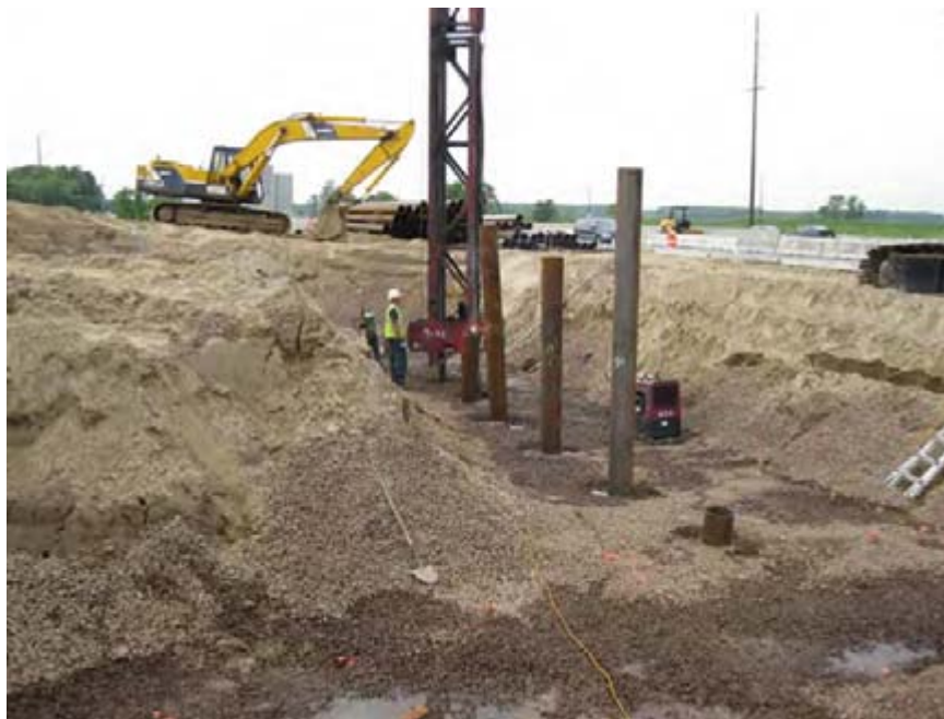
R.R. Schroeder workers driving pile for the east abutment
