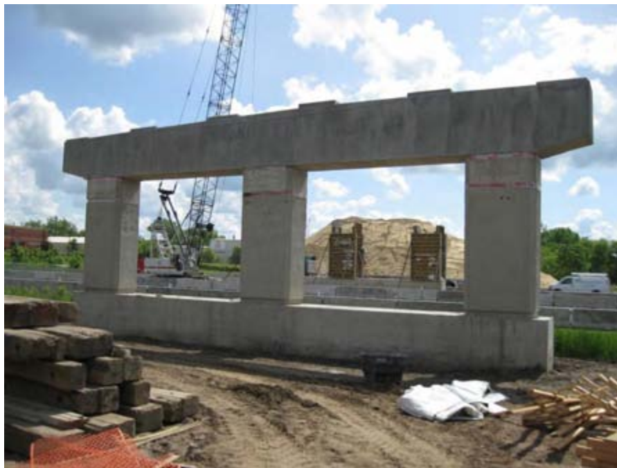
Pier 2's finished cap section
