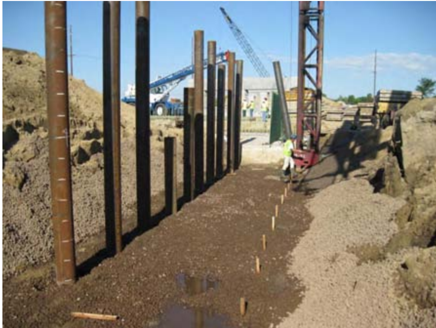
R.R. Schroeder workers driving pile for the north retaining wall
