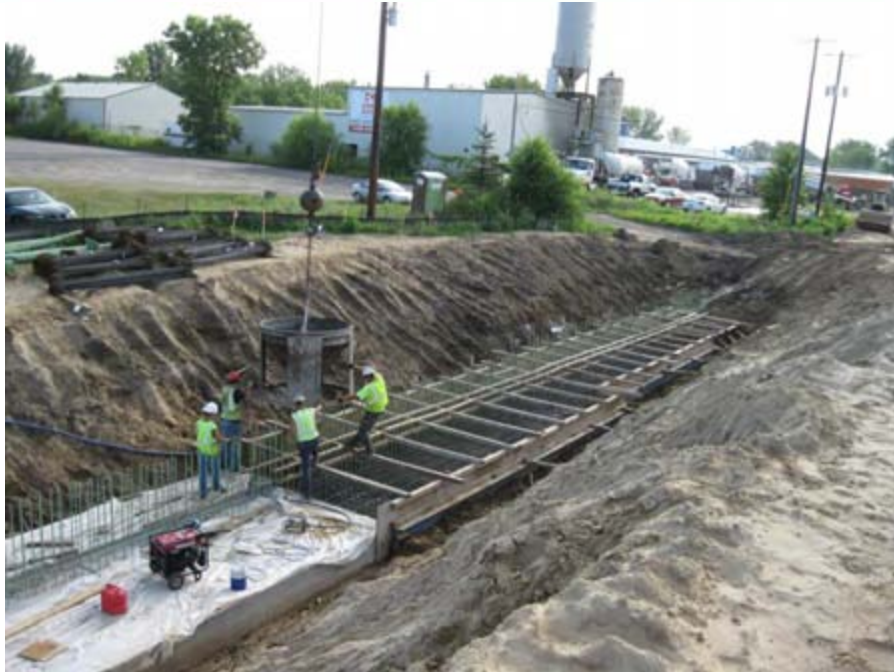
Concrete pour for panels 5, 6, and 7 footings of the north retaining wall
