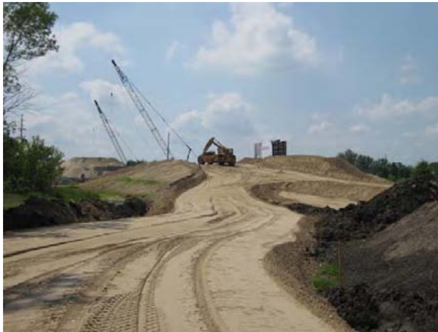
Excavation of the east surcharge
