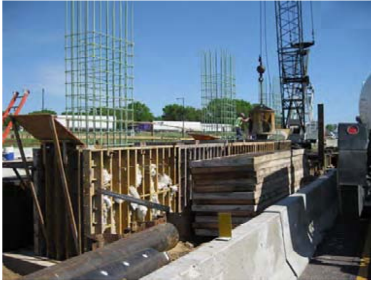
R.R Schroeder workers pouring pier 3's crash strut.
