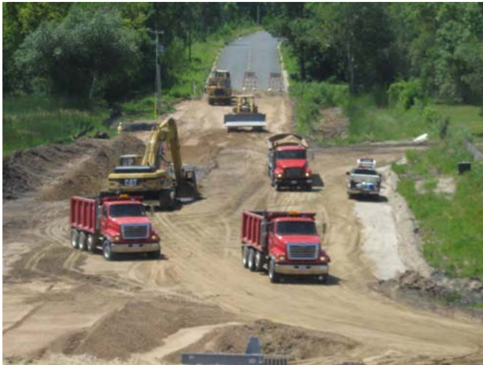
Forest Lake Contracting muck excavating on CR 83
