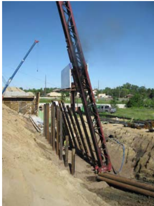
Pile being driven for the north retaining wall
