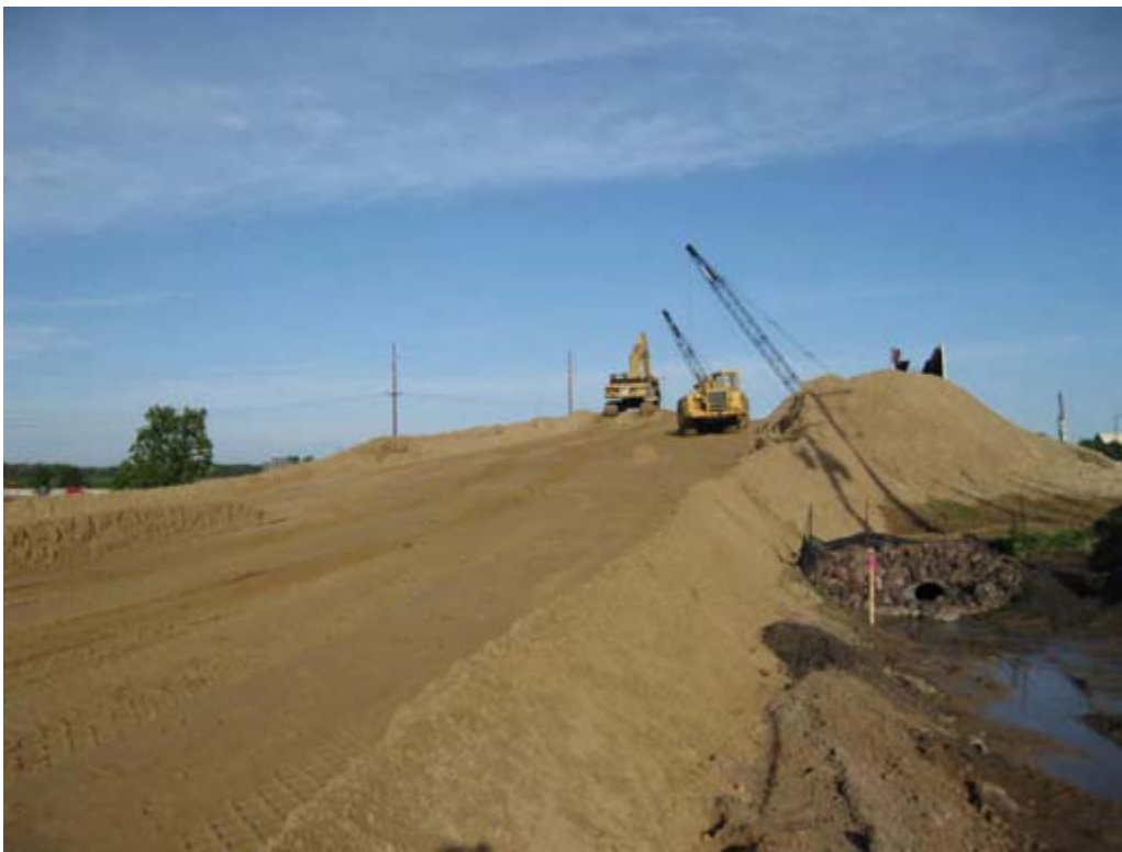
Removal of embankment material on the east surcharge
