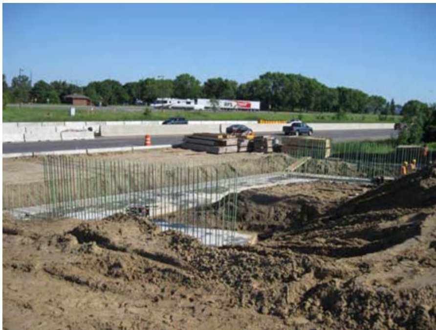
The completed east abutment footing
