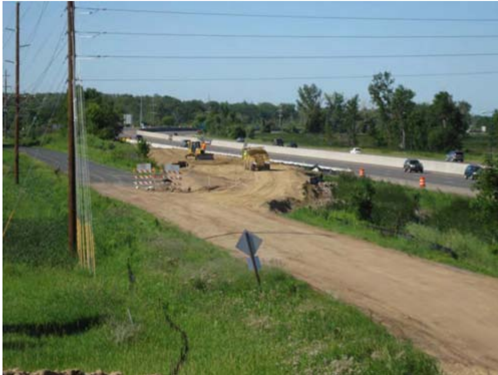
Construction of the second lift of the temporary northbound off-ramp surcharge
