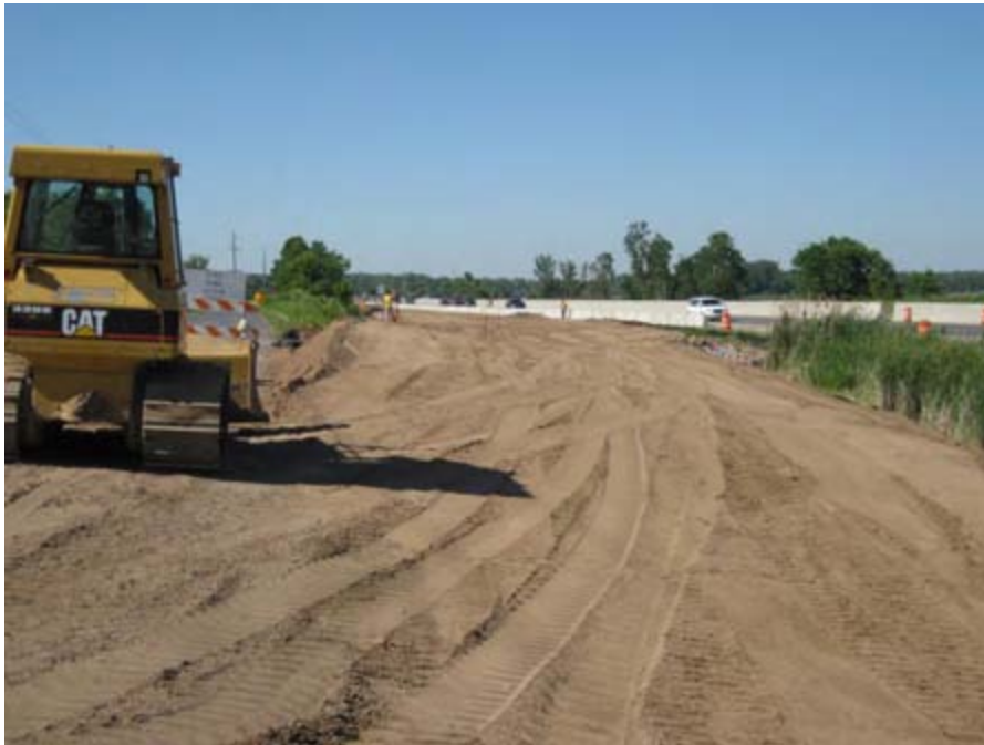
Temporary northbound off-ramp surcharge after placement of 1 st lift
