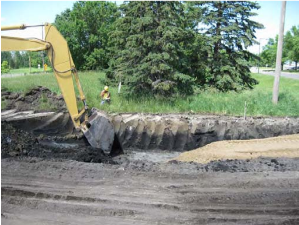
Subcutting followed by granular backfill on the Mn/DOT haul road
