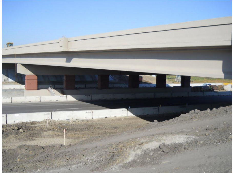
A look at the newly painted bridge
