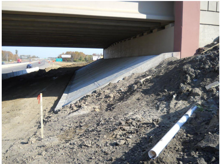
A look at the completed east abutment slope paving
